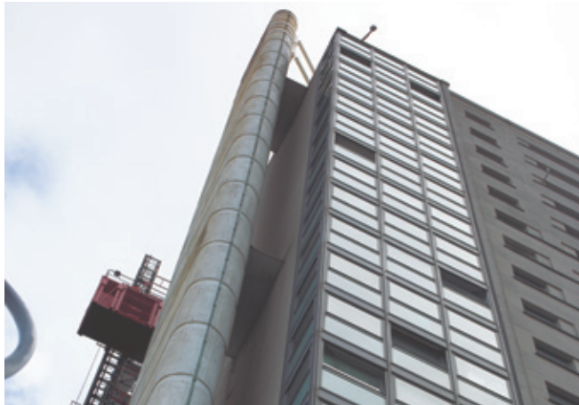
Existing flue fixed to the side of Seaton Point
