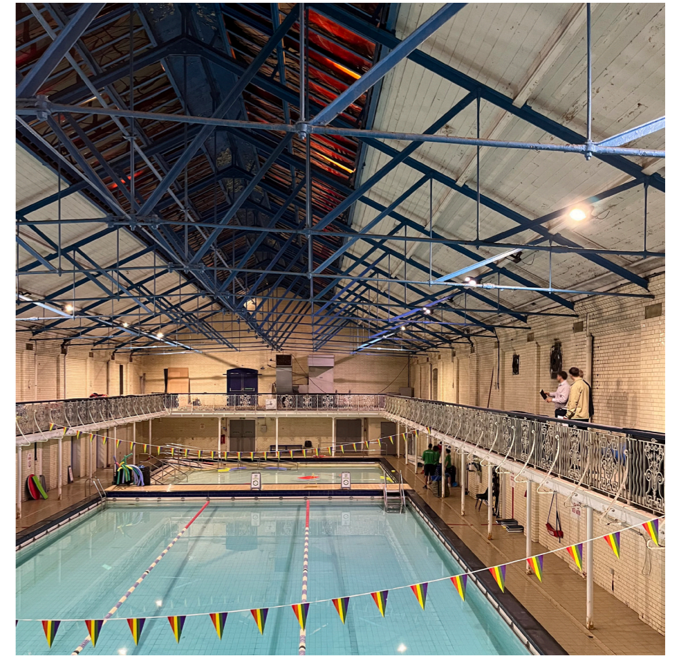
Existing Mixed Pool - Former First class Males Pool
