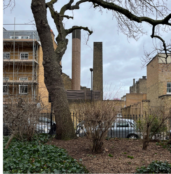
Existing boiler house to Clapton Square
