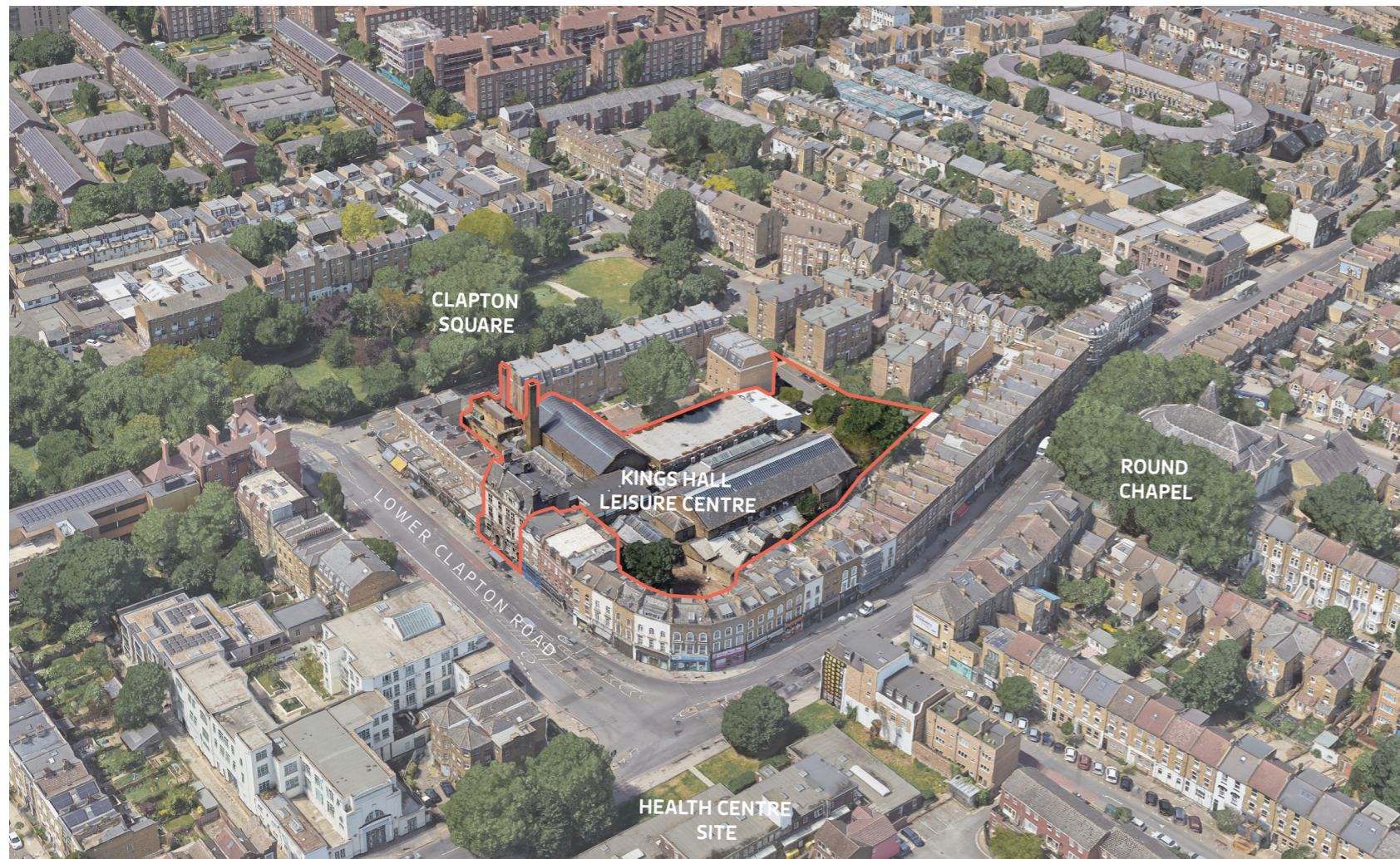
Aerial View of Existing Facility
