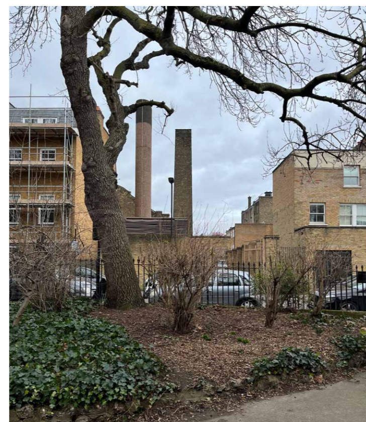
Existing boiler house to Clapton Square
