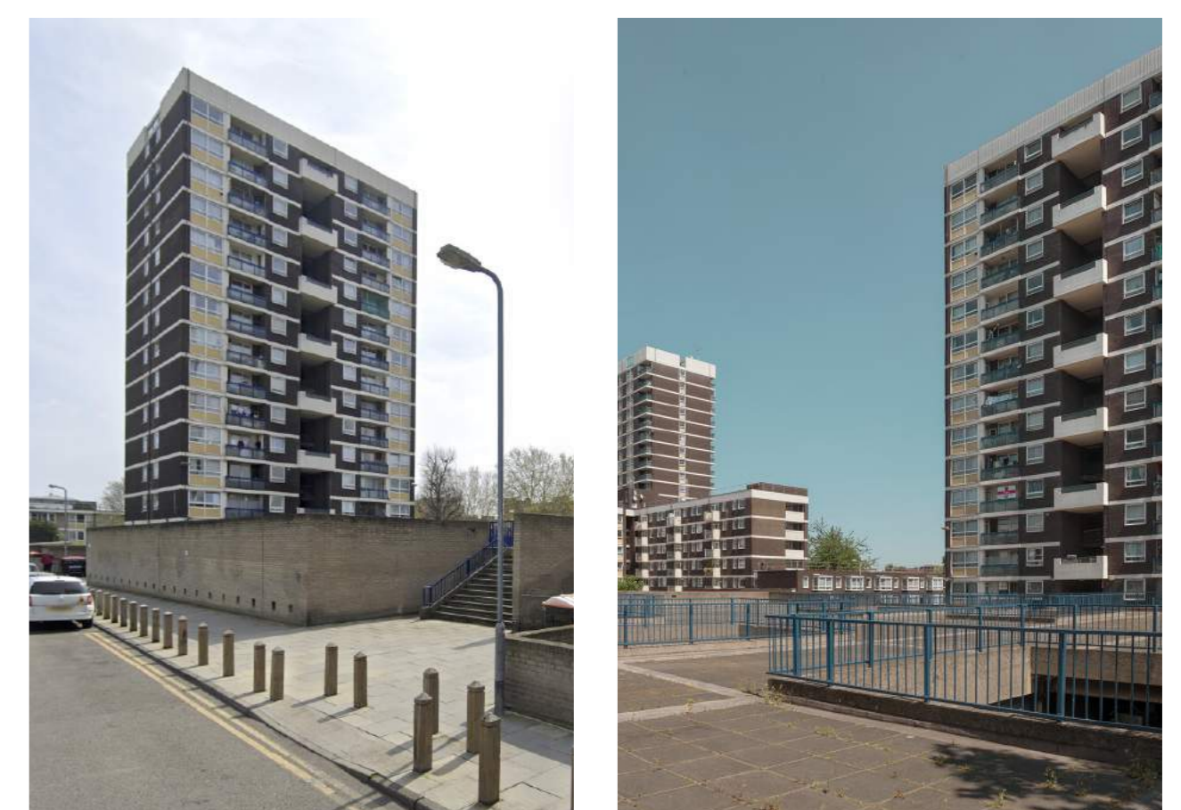
F) Views of the existing parking podium at Balmes Road
