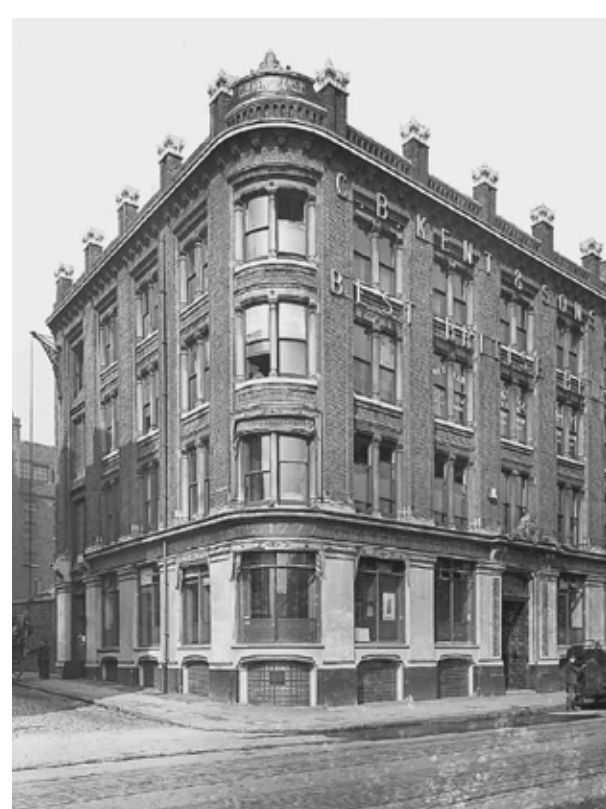
Paired windows to the apartments with an expressed roof and first floor cornice
