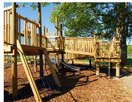
Existing timber climbing frame retained and connected to the mound via a net bridge
