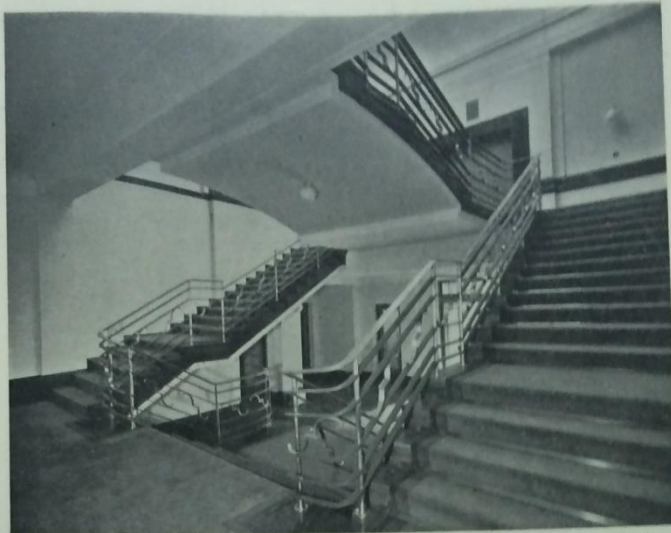
The teak stair leading to the council suite. The balustrade is in wrought iron and silver bronze.
