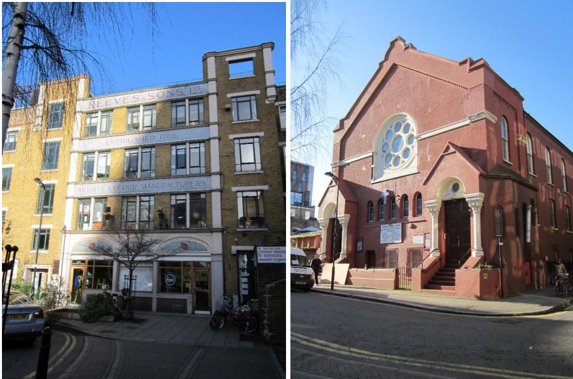
Figure 25 & 26: Nos. 18-22 Ashwin Street and the Shiloh Pentecostal Chapel
