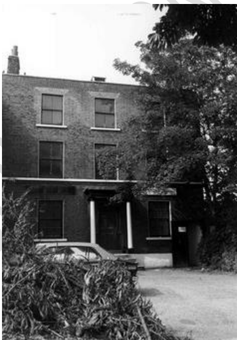
Figure 20: No. 57 Dalston Lane
