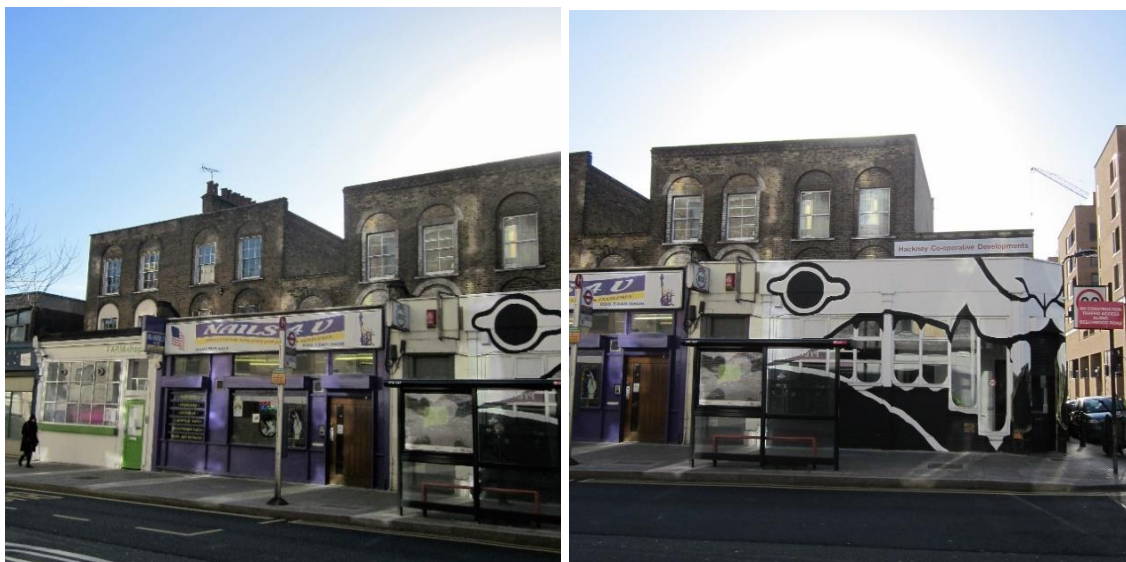
Figures 28 and 29: Nos. 16-20 Dalston Lane
