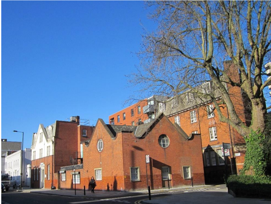
Figure 13: The former Police Station and residential annex behind
