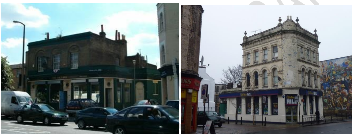
Fig. 23 & 24 :The Victoria Public House, No. 451 Queensbridge Road and the former Railway Tavern at No. 11 Dalston Lane in 2011
