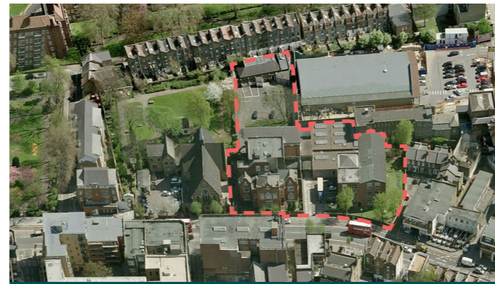
Existing aerial view from west
