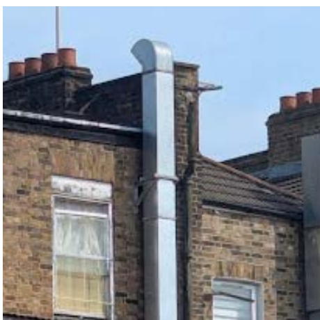
✓ Figure 3.4 – Example of simple acceptable ducting usually seen to the rear of a commercial building.
