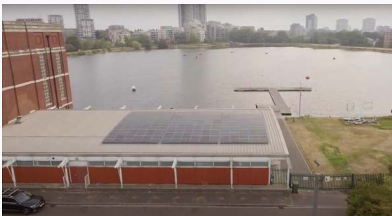
✓ Figure 3.8 – Hackney Light and Power – The solar panels, installed at the West Reservoir Centre by Spirit Energy, are set to generate 77,000kWh of power per year, covering all of the centre's electricity needs. The PV panels are located away from the edges of the roof.
