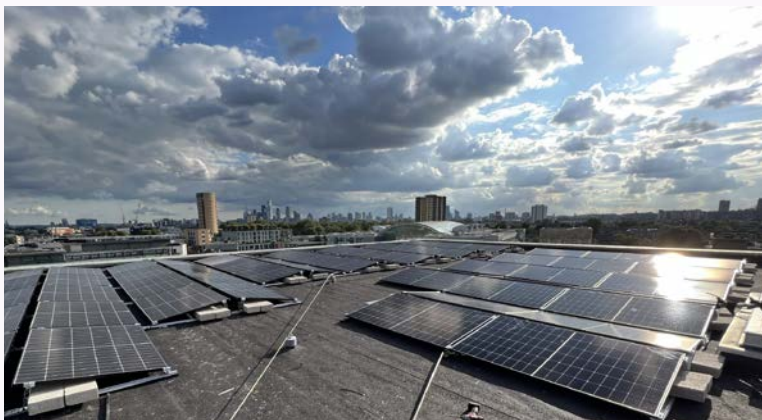
✓ Figure 3.7 – Hackney Empire Grade II* listed PV's located in the middle of the roof and not noticeable from the street or surrounding buildings. (Photo Credit Hackney Light and Power)
