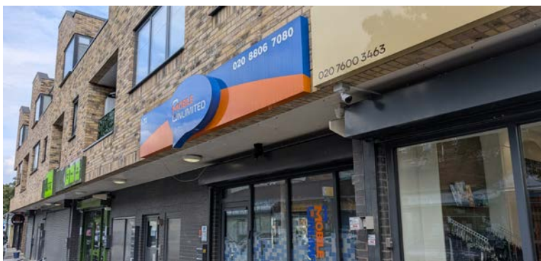
✕ Figure 5.10 – A contemporary shopfront with limited space dedicated to signage, a lack of practical traditional elements such as stallrisers, and prominent security shutter boxes. Signage is placed above the fascia at different heights, creating a cluttered appearance.
