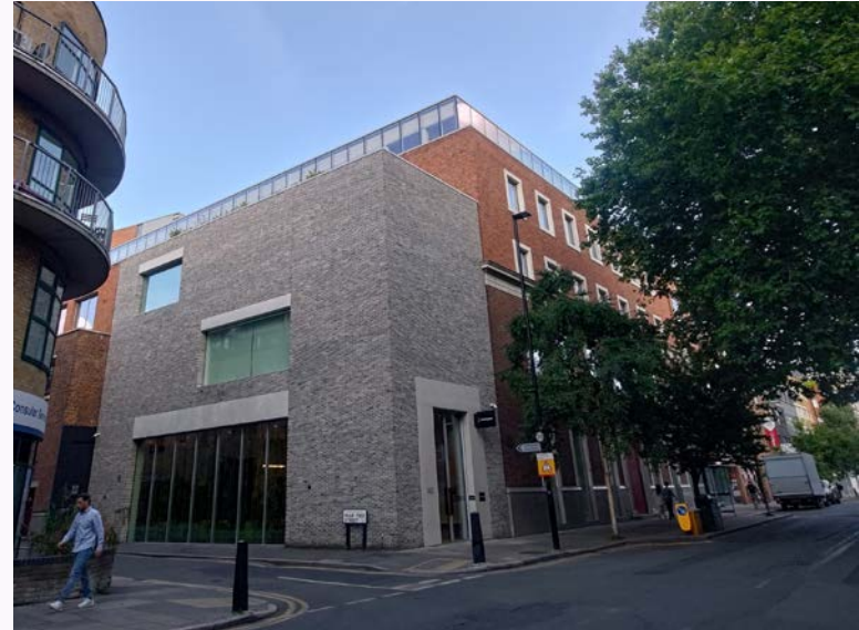
✓ Figure 2.7 – A three storey timber framed office extension to a former distillery, including two storeys of matching window and brick and one glazed storey.
