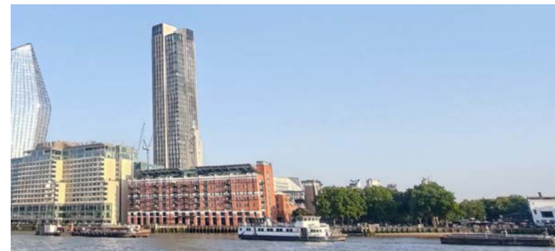
✓ Figure 2.11 – This tower, in an area considered suitable for tall buildings, has been extended by thirteen lightweight storeys. The entire building has been refurbished in a consistent style to create a cohesive whole.
