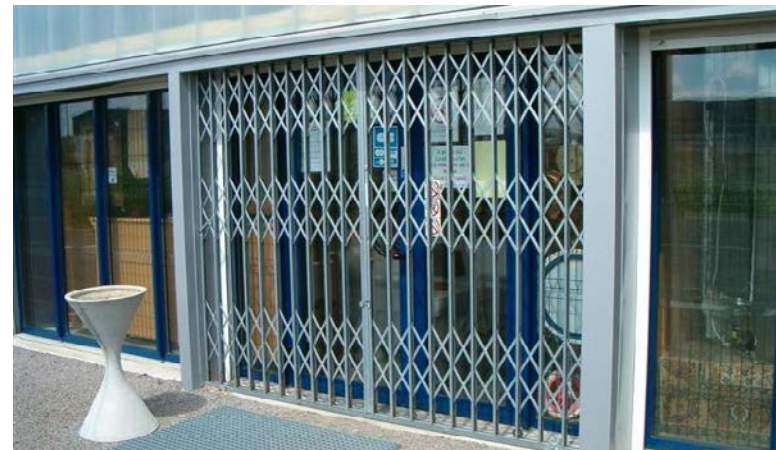
✓ Figure 5.14– A contemporary external grille, powder coated to match the overall colour and design of the shopfront.
