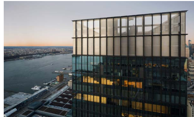
✓ Figure 3.1 – Rooftop plant surrounded with a semi transparent mesh screen as a considered part of the architecture.
