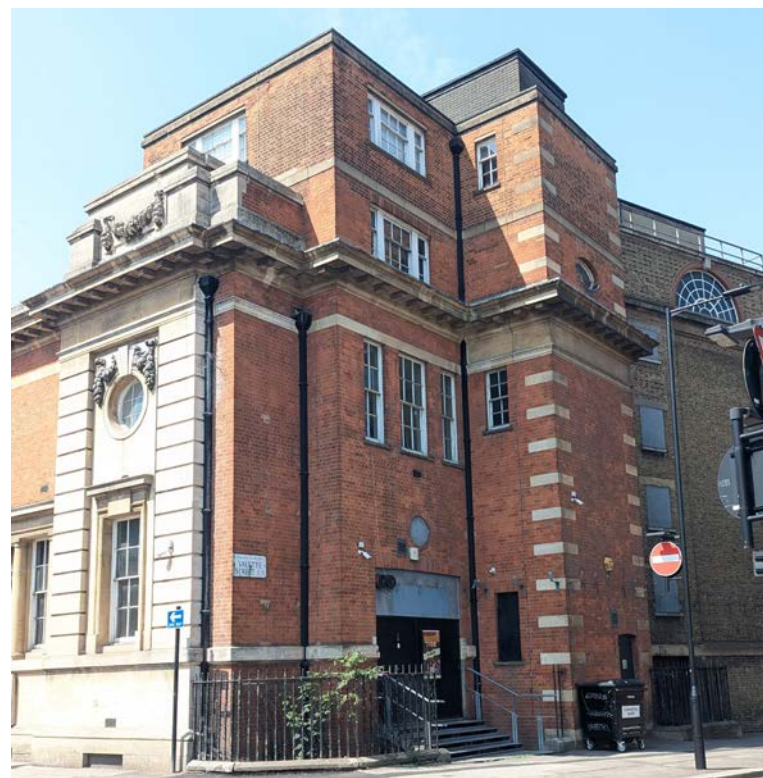
✓ Figure 3.5 – Continuous integrated gutters placed at the corners of the building and made out of powder coated metal.
