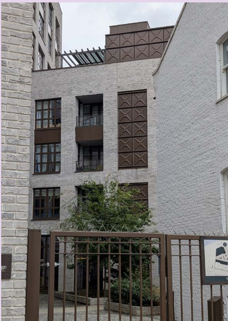
Figure 3.2 – Visible rooftop plant enclosure designed as an integrated part of the architecture.
