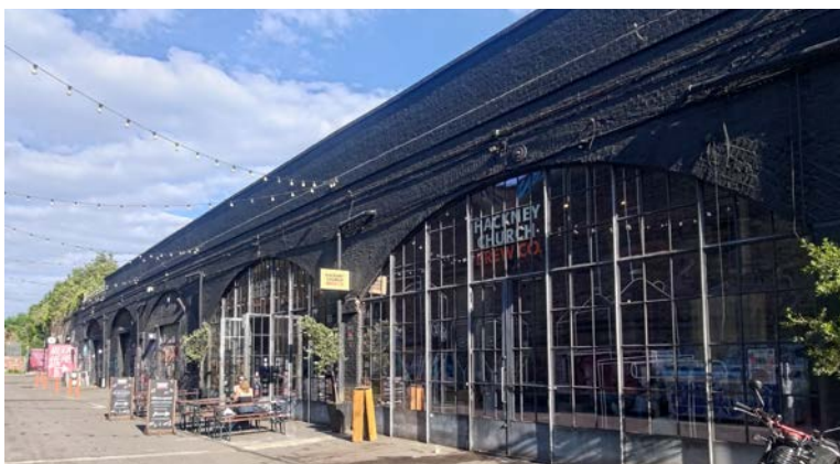
✓ Figure 5.12 – A good quality modern retail frontage within a railway arch that maintains the overall form and opening size.
