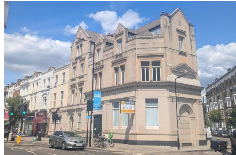
✓ Figure 2.10 – Some buildings are unsuitable for upwards extensions. This historic building is a complete architectural composition in an area of consistent height where an extension would have a negative impact on the roofscape.
