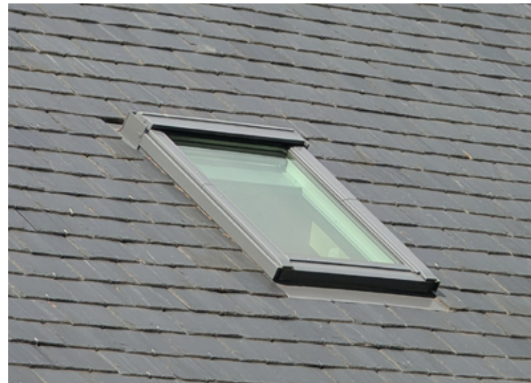
Figure 6.21 – Standard roof light projecting from the plane of the roof.
