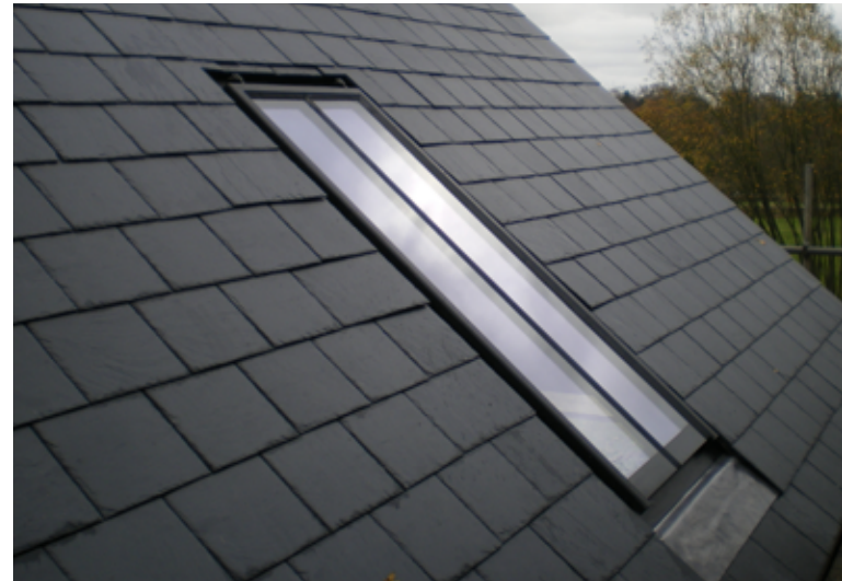
Figure 6.20 – Conservation style roof light flush with tile or slate roof covering. (Photo credit Clement Window Group )
