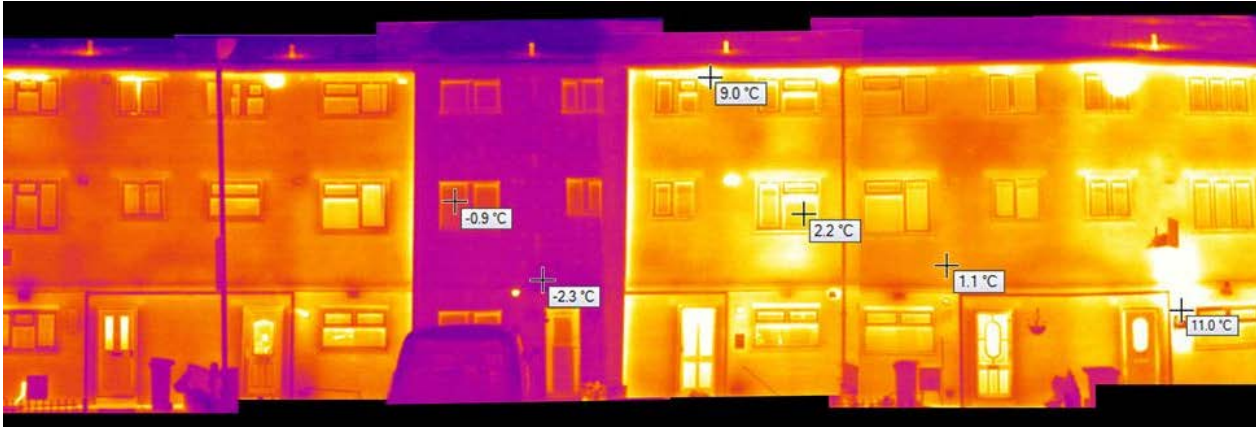
Figure 3.2 – Thermal imaging of a retrofitted home showing significant improvements to reducing heat loss in a terrace. The property with retrofit shown clearly in purple 'low heat loss'. (Photo Credit: bere:architects)
