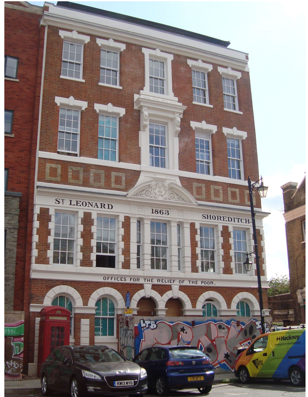
The facade of St Leonard Parish Relief Offices has been refurbished as part of a regeneration project for the wider hospital site
