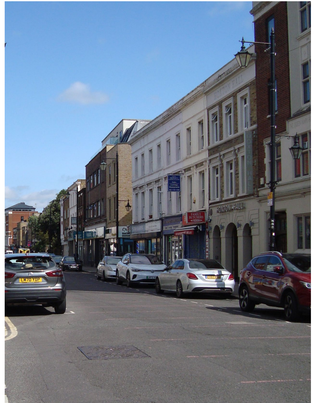
View of Hoxton Hall and the heart of the Hoxton Street Conservation Area looking north
