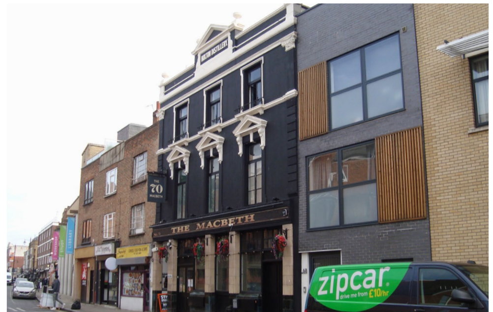
Macbeth Public House, 70 Hoxton Street (locally listed)
