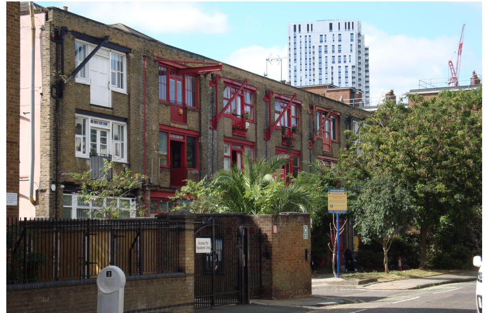
1-7 (even) Academy Buildings, Fanshaw Street
