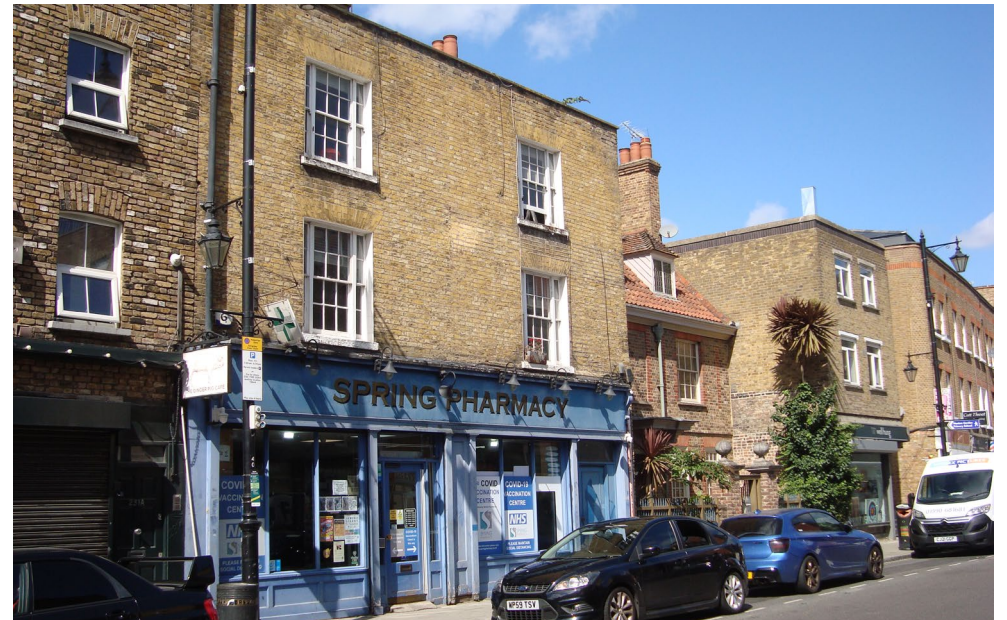
Grade II listed Nos 233 and 235 Hoxton Street, with 237 Hoxton Street beyond
