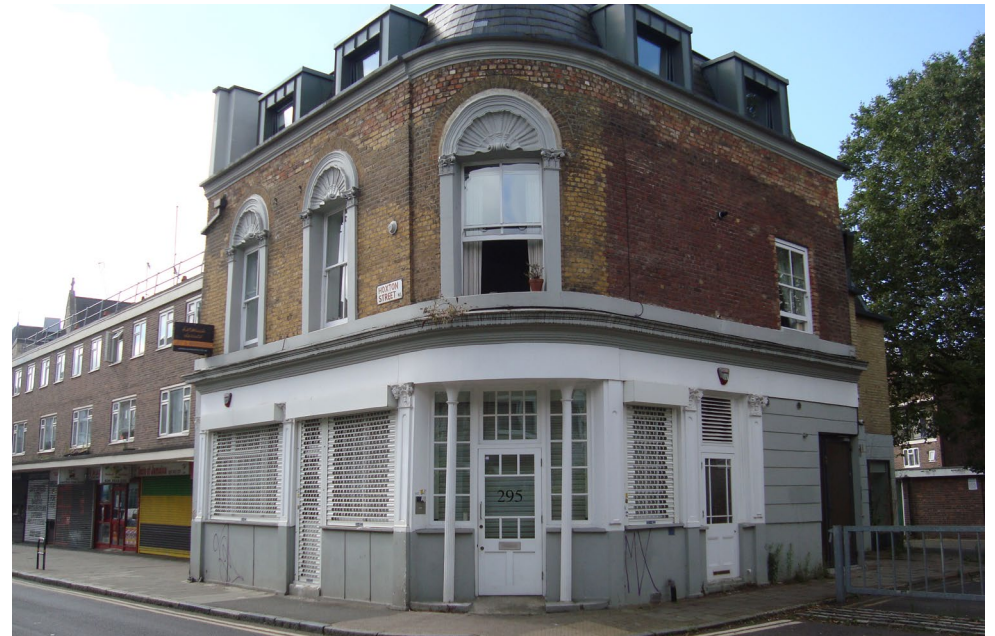
Former King's Arms pub at 295 Hoxton Street, now in residential use
