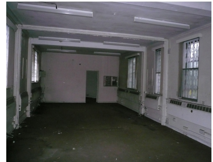
Interior of Civil Defence building
