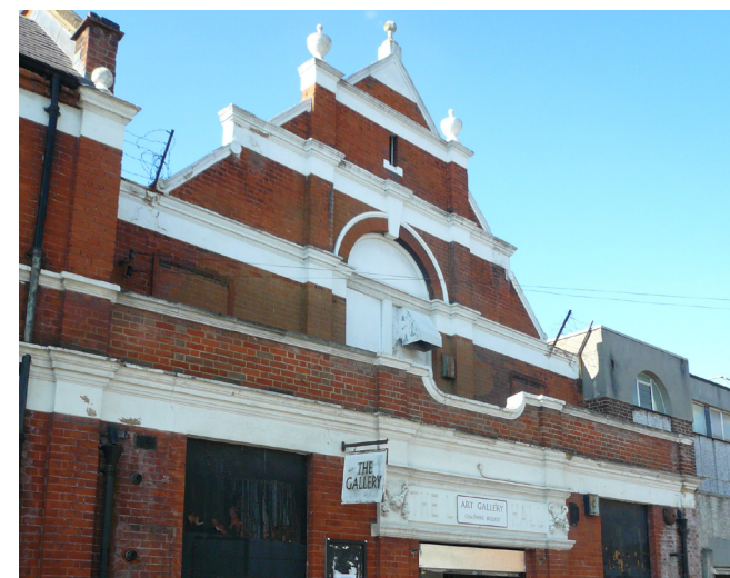
The Gallery entrance (Edward's Lane)
