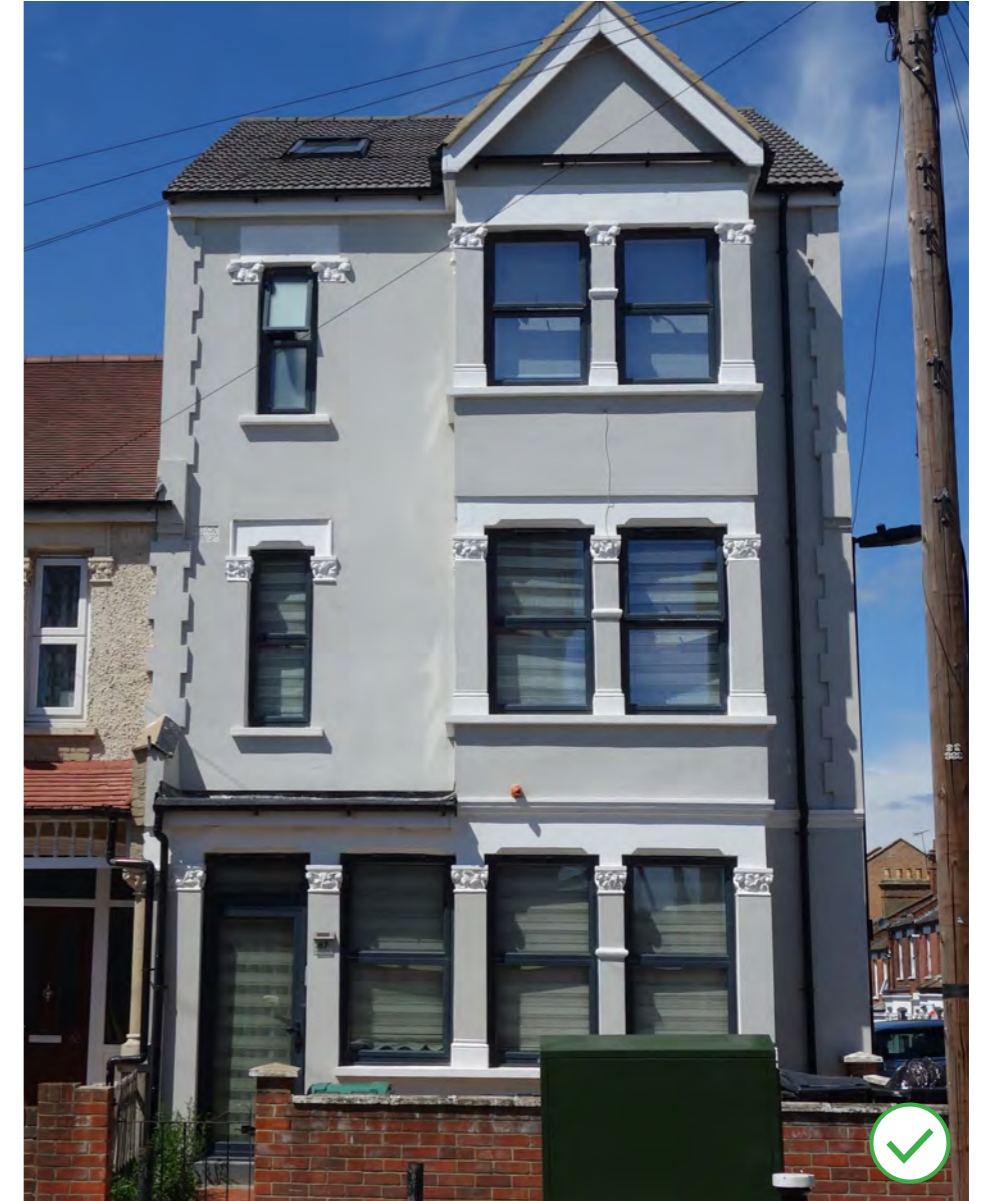
Fig.22: The additional floor level is proportional in scale and height to the existing floor to ceiling heights of the floors below
