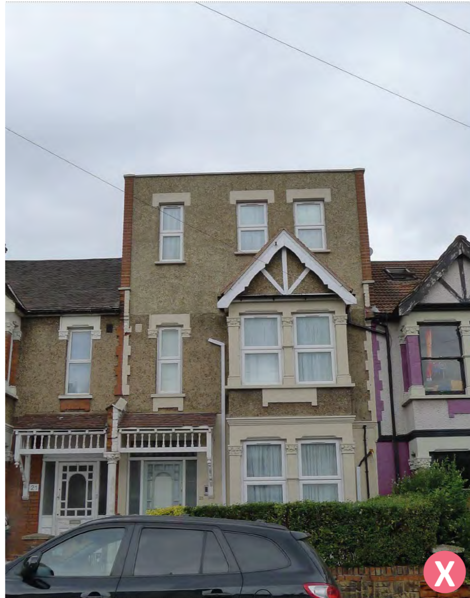
Fig.19: Roof extension has a bulky appearance and no relationship to the existing form; loss of architectural character of the existing front dormer
