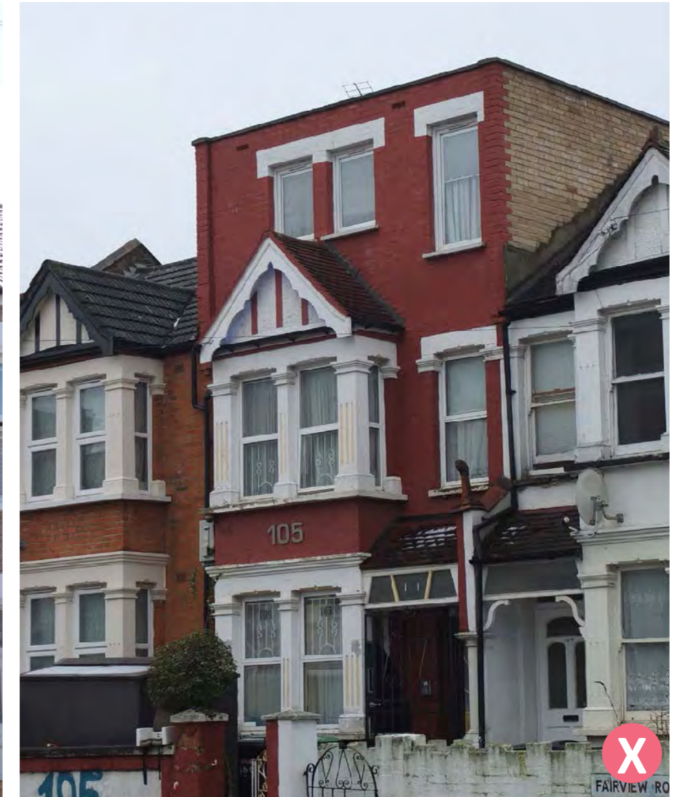
Fig.36: The roof extension is bulky and detracts from the front gables architectural character. The pitched roof form has been lost and the flat roof is not in keeping with the neighbouring properties.
