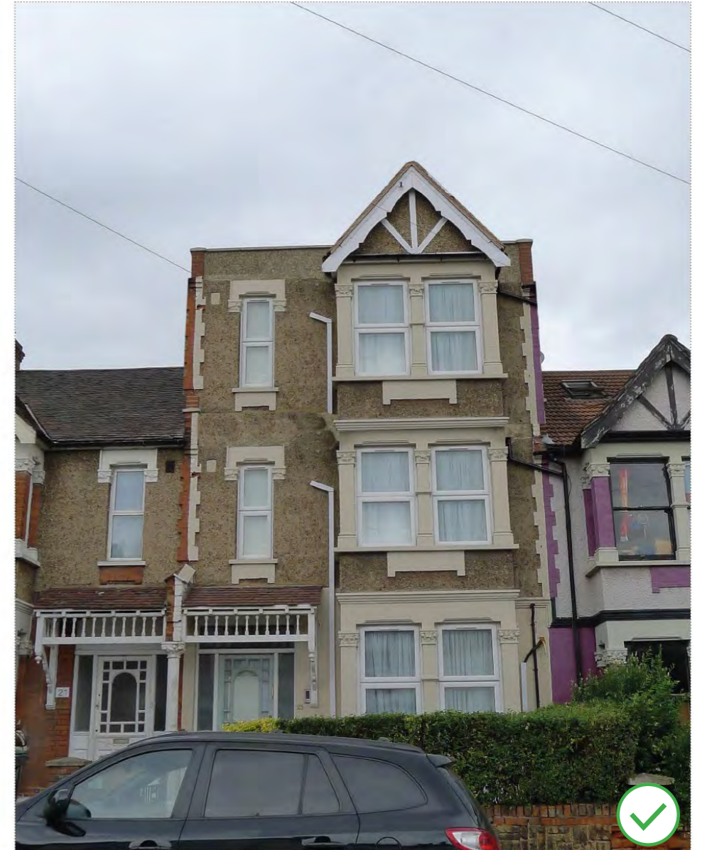
Fig.20: The characteristics of the front dormer are retained by replicating and elevating the original front dormer
