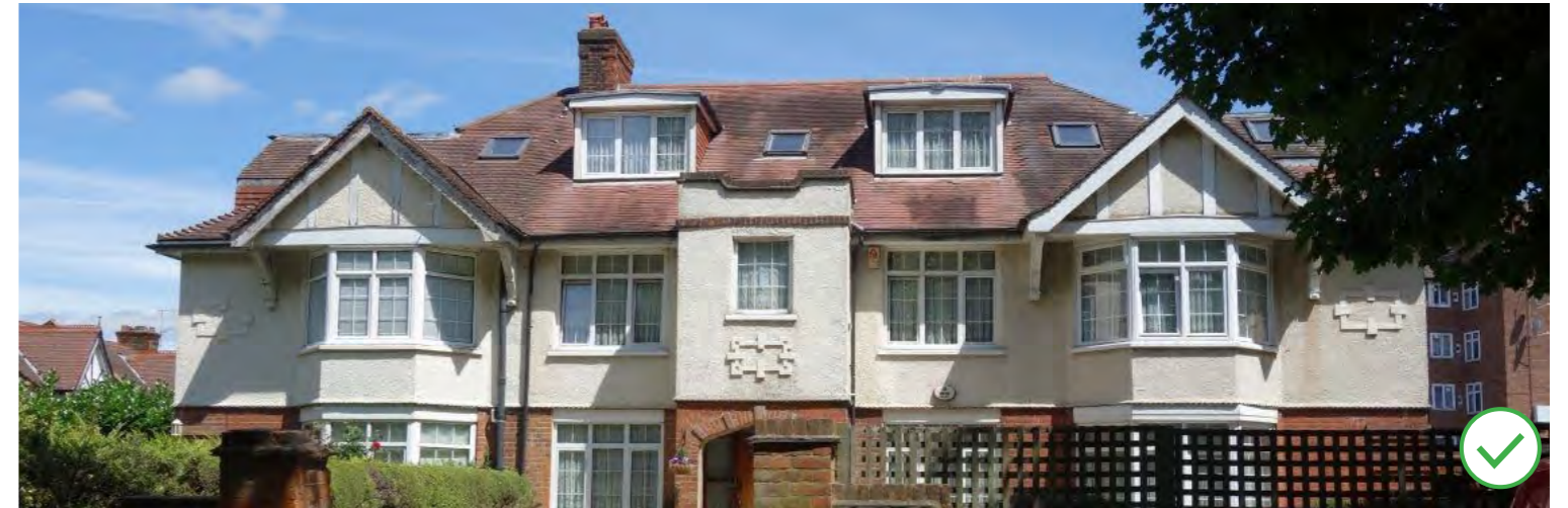
Fig.25: Acceptable dormer windows
