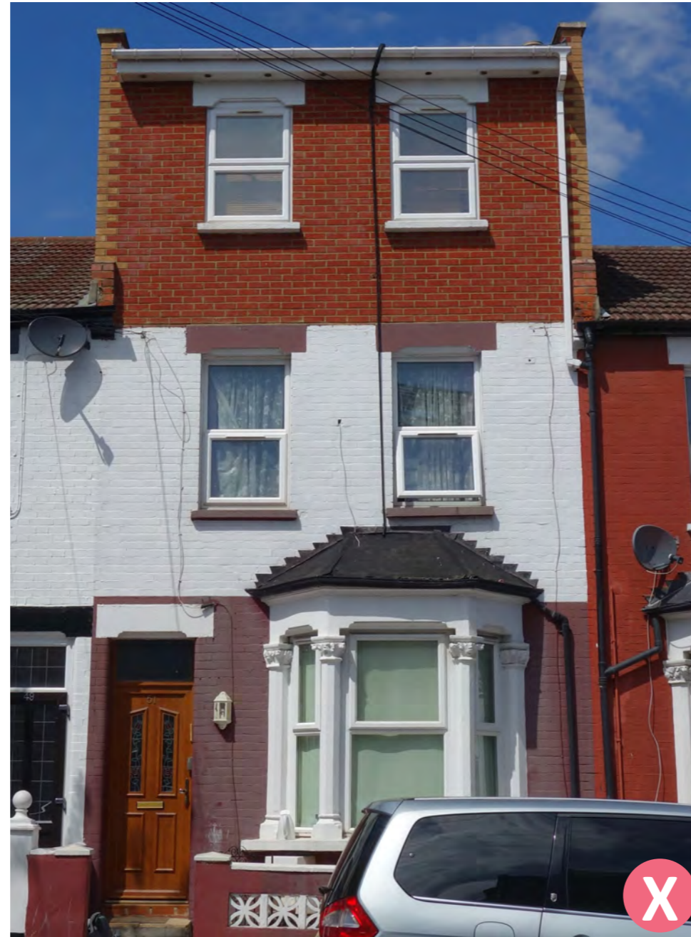
Fig.28: Roof extension is not acceptable due to change in materials that draws too much attention on the upper element
