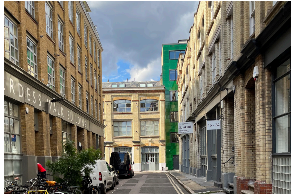
Underwood Street looking north
