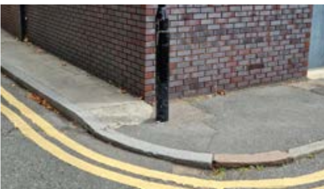
Lamp post interrupting narrow footway with missing dropped kerb
