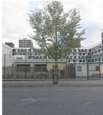
2 81 Downham Road (temporary school)
