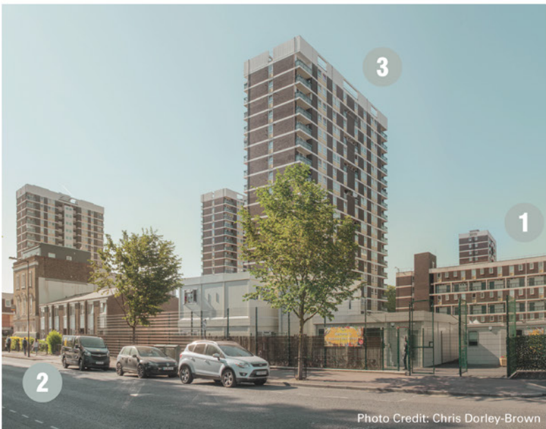
(1) Horizontal blocks, (2) Row houses and (3) Towers all have a consistent character made by the brown bricks and exposed concrete slabs
