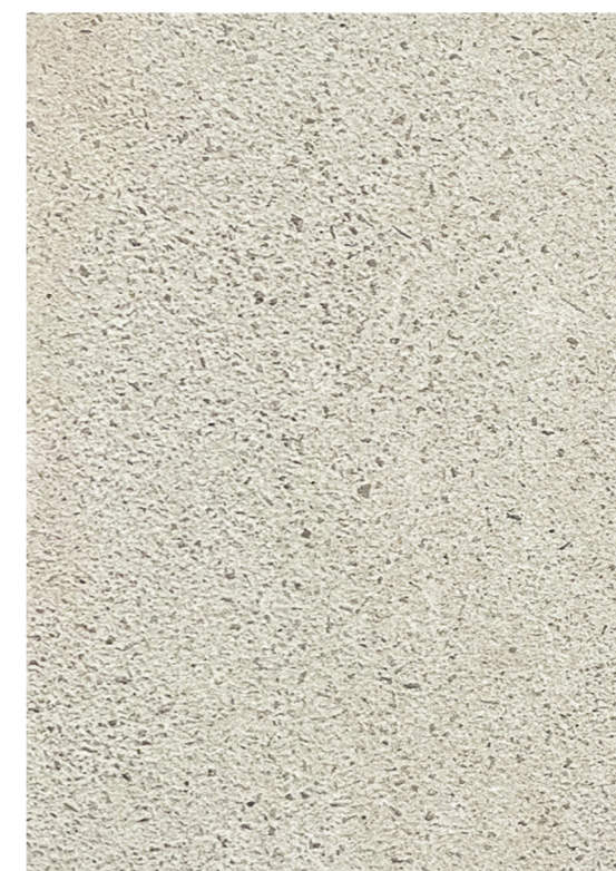
Precast concrete spandrel panels and string coursing
