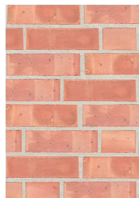
Brickwork - External gallery wall
