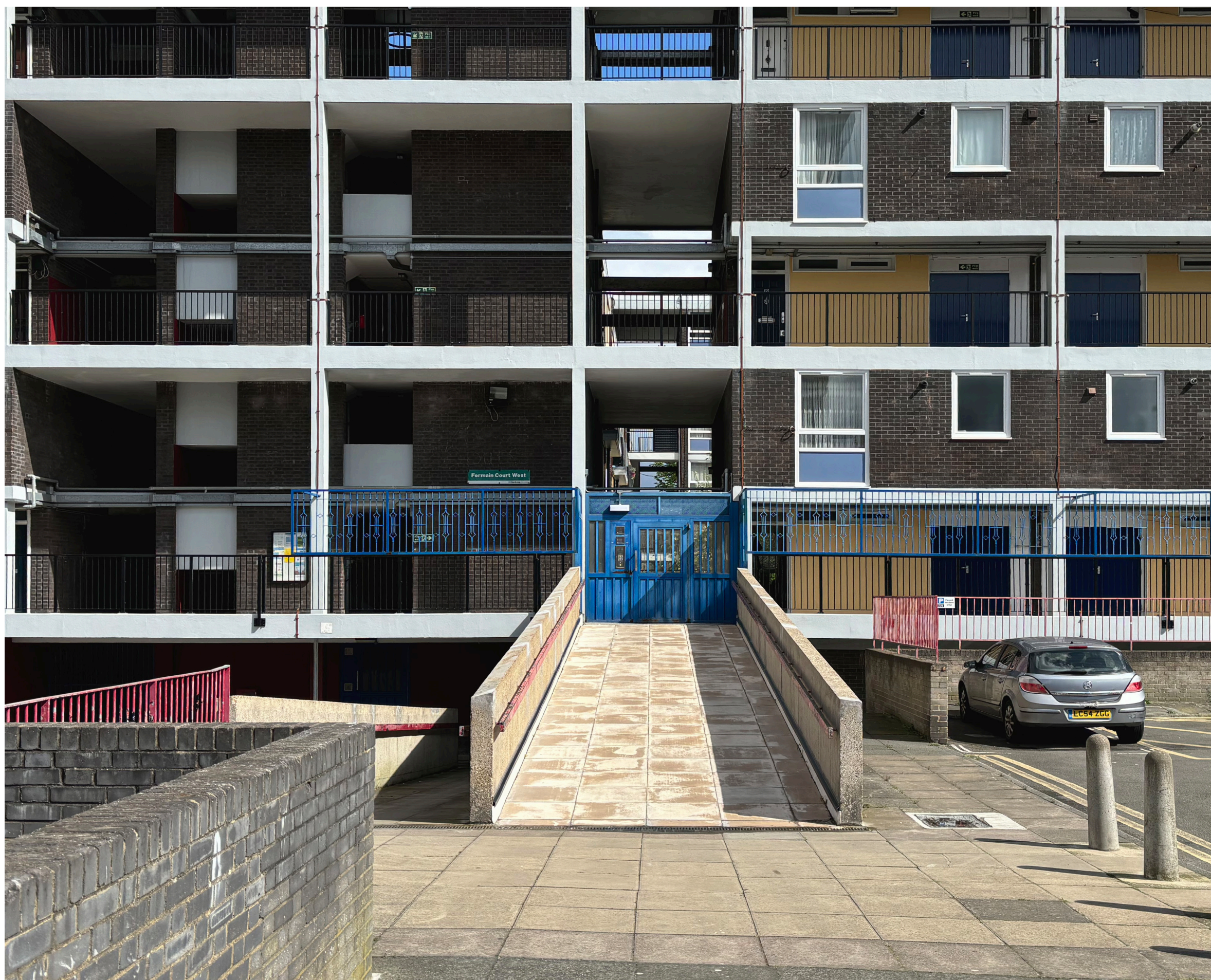
Existing Fermain Court Western Entrance
