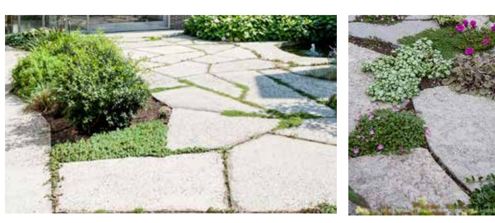
03 The upper level of the garden is at street level to allow existing shortcuts to continue through. We propose using the existing concrete, with some sections broken up to allow plants to self seed.
