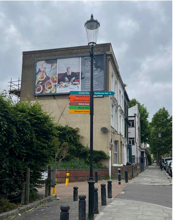
Directional signs clamped to existing lamp post
