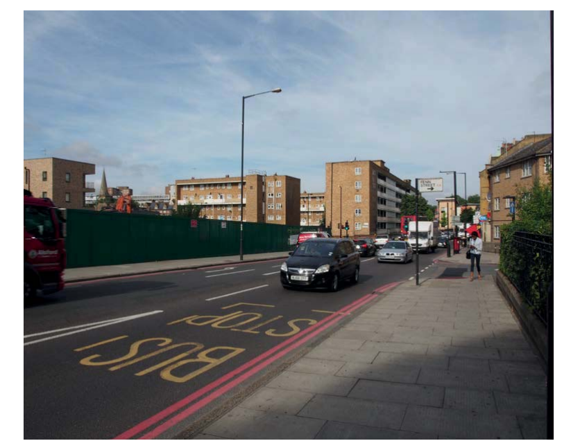
Marian Court pre-demolition
