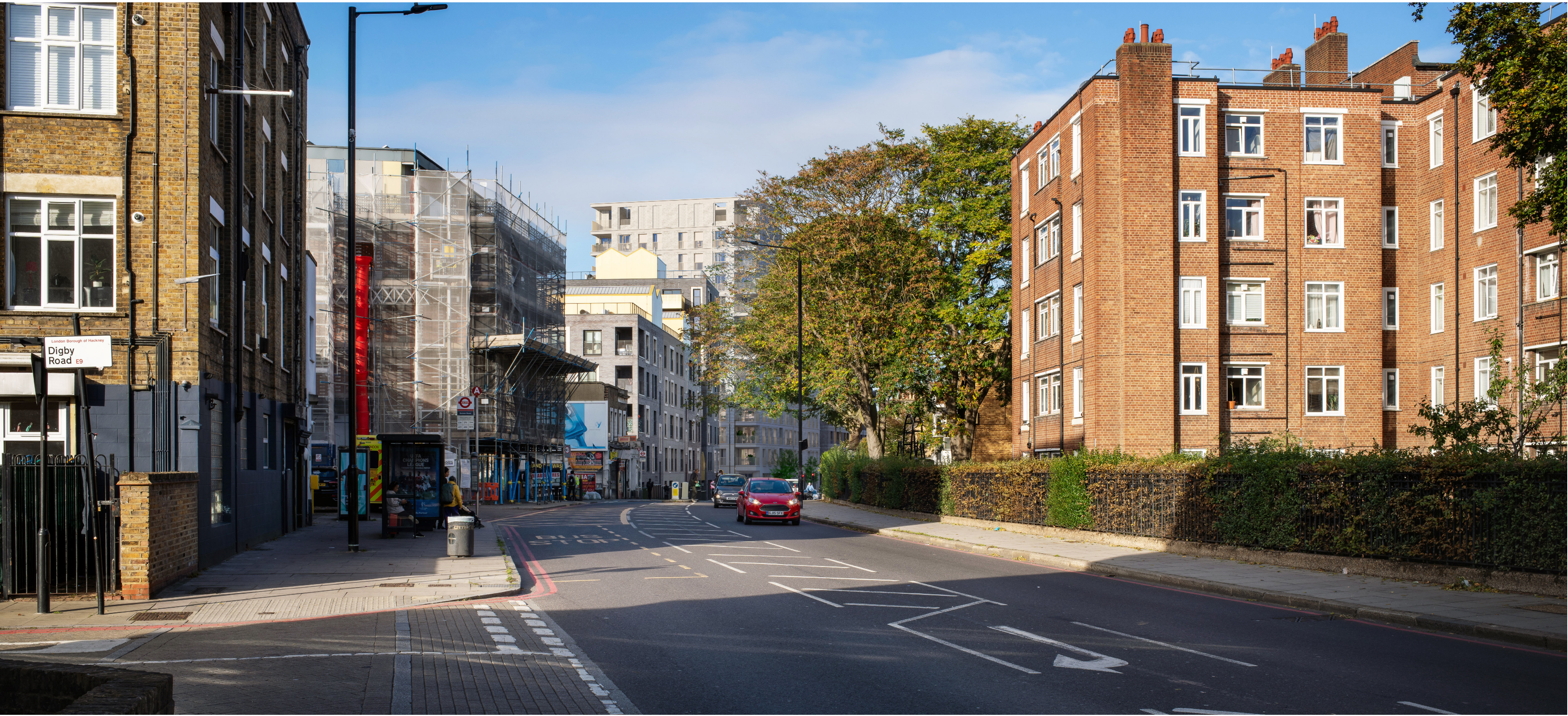
View west along Homerton High Street
