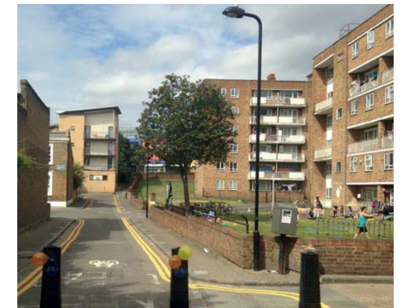
Marian Court pre-demolition
