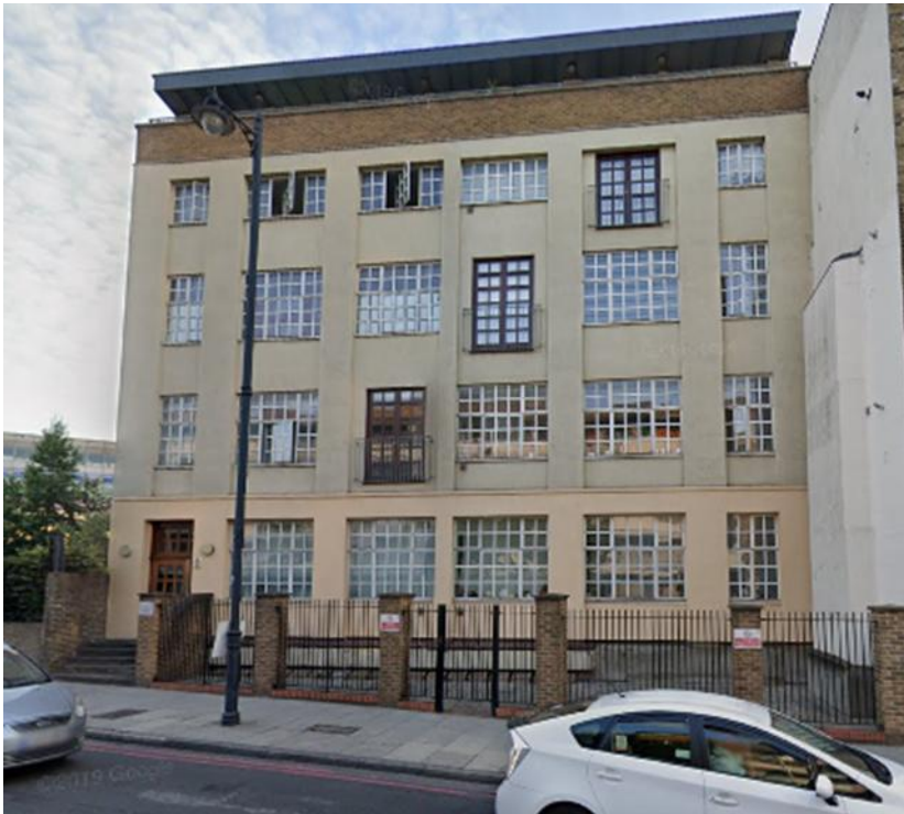
Image 5 - Street View of 17 Homerton High Street, southern elevation
