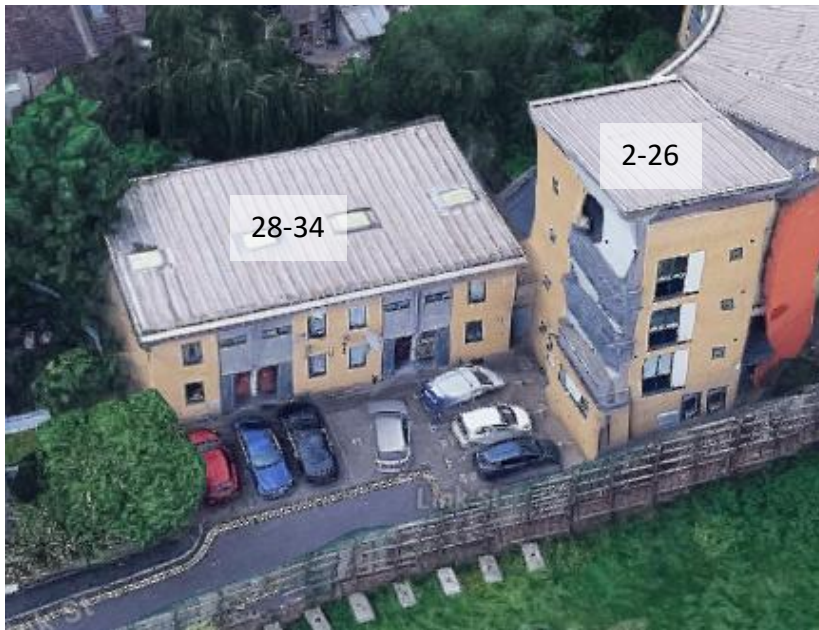
Image 4 - Aerial view of 2-26 & 28-34 Link Street, Eastern and Southern elevations
