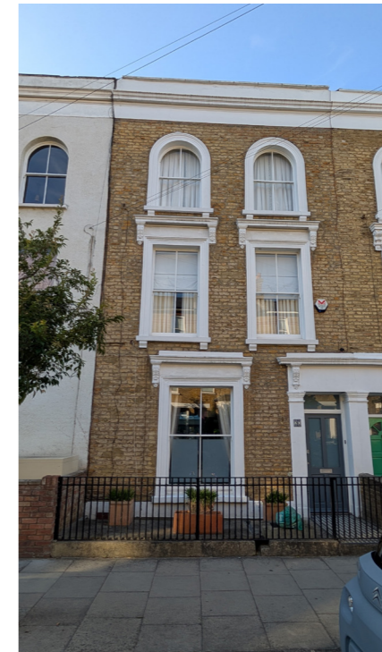
C: Staggered windows, arched windows higher up, detailed parapet
