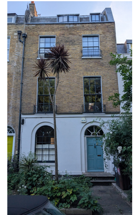
D: Rendered base, slightly recessed frame around ground floor openings.
