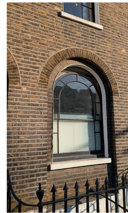
Arched window to ground level
