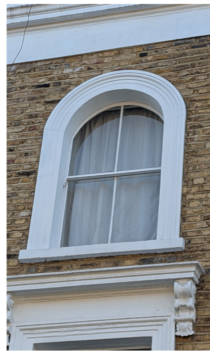
Arched window on upper level
