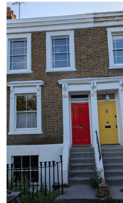
G: Staggered windows, white semi-basement, white frames around openings, detailed parapet
