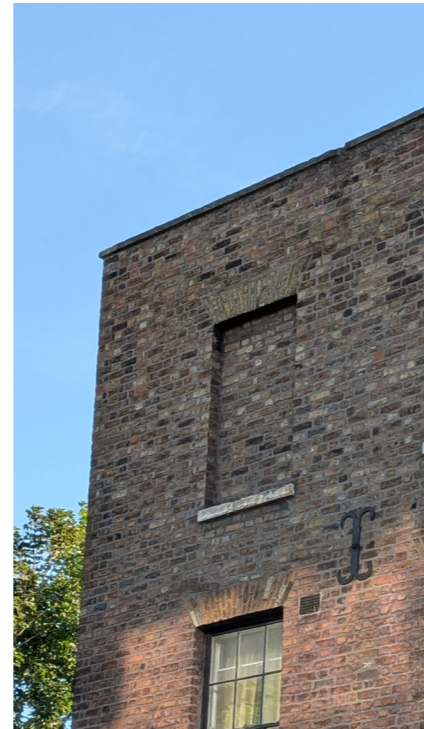
Filled in window openings
