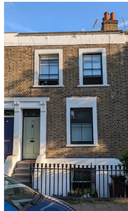
F: Staggered windows, white semi-basement, white frames around openings, plain parapet
