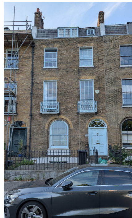
E: Staggered openings, decorative brick lintels, strong arched windows to ground floor, curved julliet balconies
