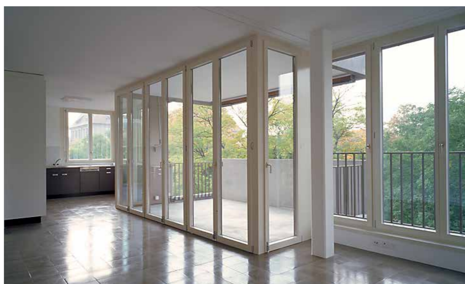
Example of an half inset balcony with a ledge outside the windows
