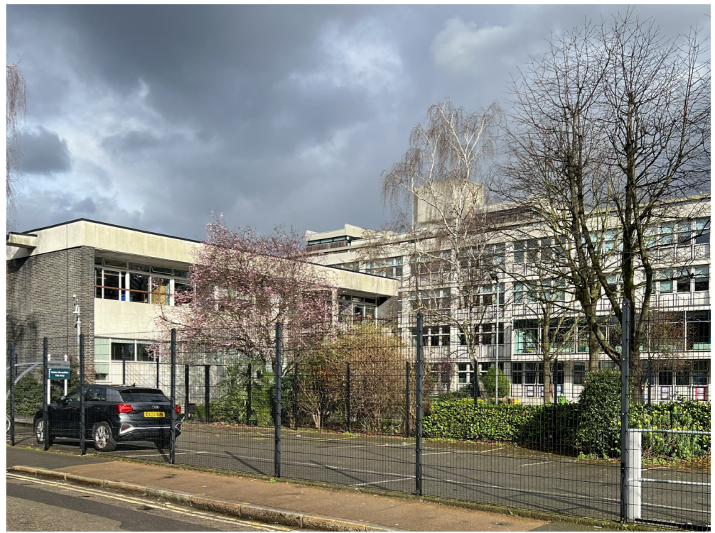
St Mary's Estate, Haggerston School is a key heritage asset within the Hackney Road Conservation Area
