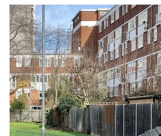
Existing example of building height variation on Fellows Court estate provides a comparison to the proposed relationship between the existing 3-storey block and new 5-storey block
