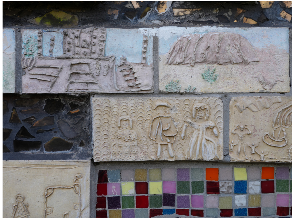
Fellows Court Community Centre, community made tiles and mosaic to the community centre and nursery entrances
