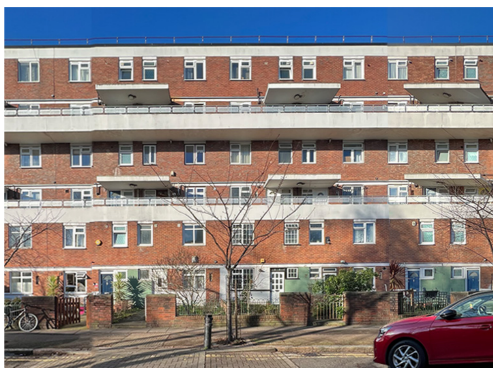
Fellows Court, linear blocks with clearly defined corners and street frontages
