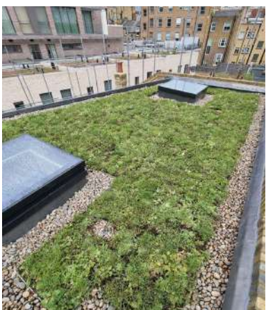
Example Green Roof
