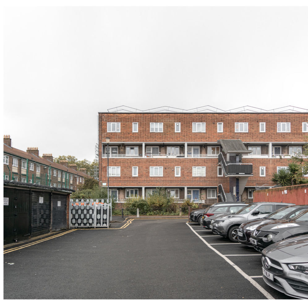
Existing garages and carparking
