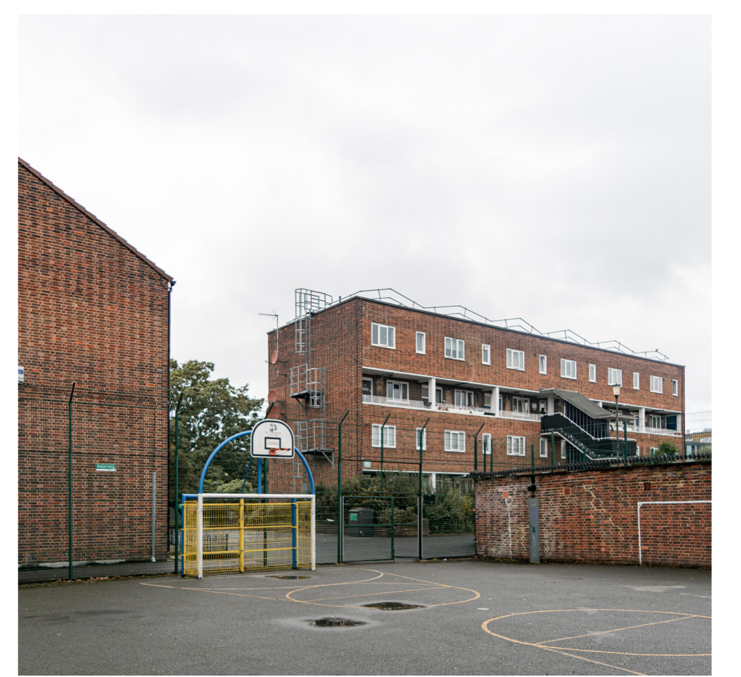
Pedestrian access along Pedro Street
