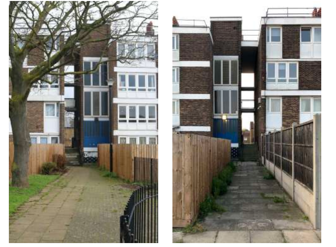
High garden fences create narrow and poorly overlooked cut throughs from Pownall Road which are current hotspots for ASB.
