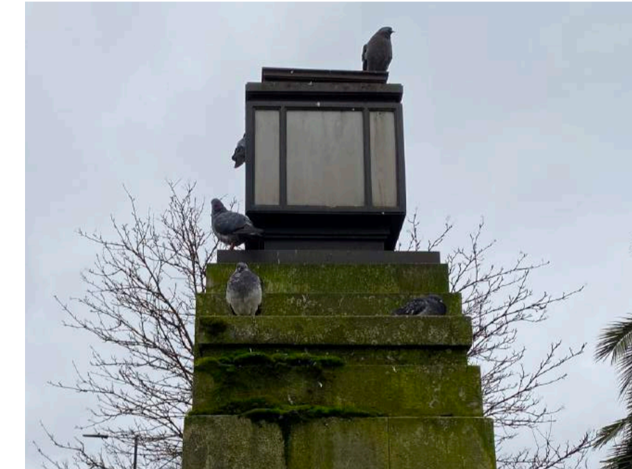
1b Cleaning the existing features, such as Town Hall Steps.
