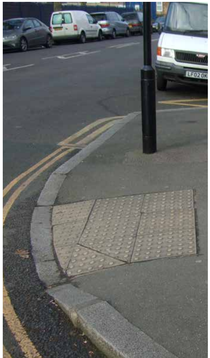
Tarmac Kerb buildout
