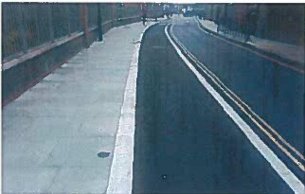
Example of a pavement and cycle track separated by a pedestrian/cycle separator
