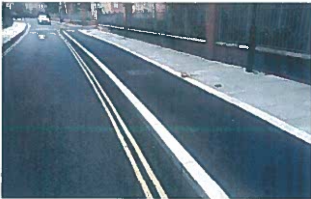
Example of a raised cycle track
