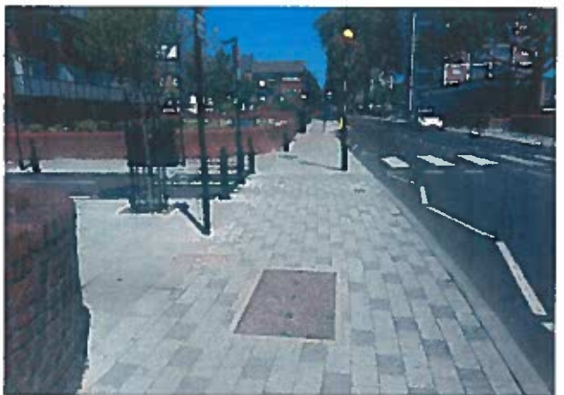
Example of a blended pedestrian crossing with a set back side road
