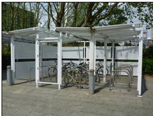
Bad practice – the siting of the door and the spacing of the stands means that those on the right cannot be used – gap between roof sections allows rain to enter
