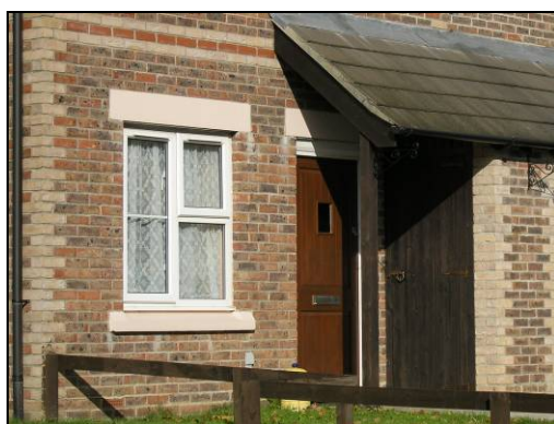
Cycle parking built into an extension of the porch: preferred approach
