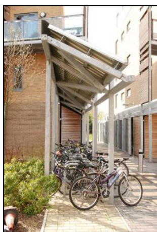
Good quality design and location of visitor parking marred by inadequate protection from the elements
