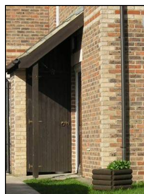
Cycle parking built into an extension of the porch: preferred approach
