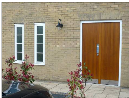
Communal (left – single door preferred unless automatically operated) and private (right) access doors to cycle parking can be both wide and attractive
