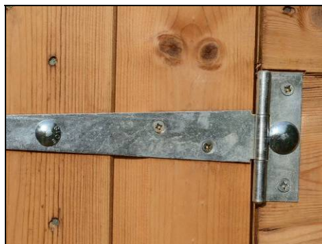
External hinges that rely on screws that can be removed from outside should not be used or additional, secure bolts provided
