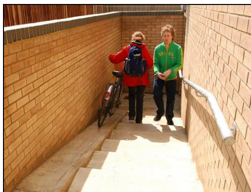
Steps and wheeling ramp giving access to communal cycle parking area (two ramps would improve ease of use)
