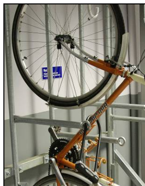
Hanging rack with means of locking the frame (not normally recommended)
