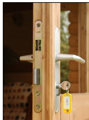
Good practice: Mortice locks provide greater security
