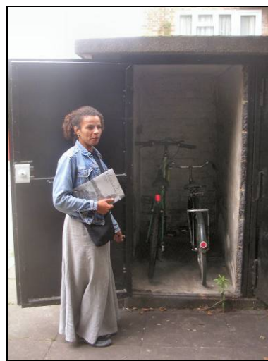
Retro-fit solution – secure doors fitted to disused pram shed
