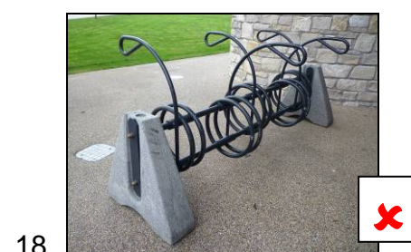
Inadequate support, potential for damage to wheel and poor security
