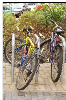
Stands too close together only leave room for one bicycle per stand
