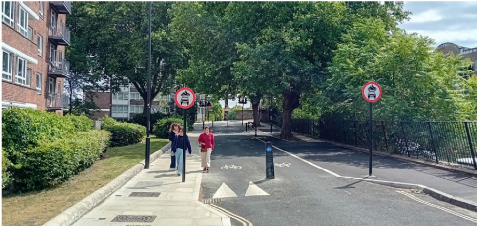
Example of a closed side road using bollards
