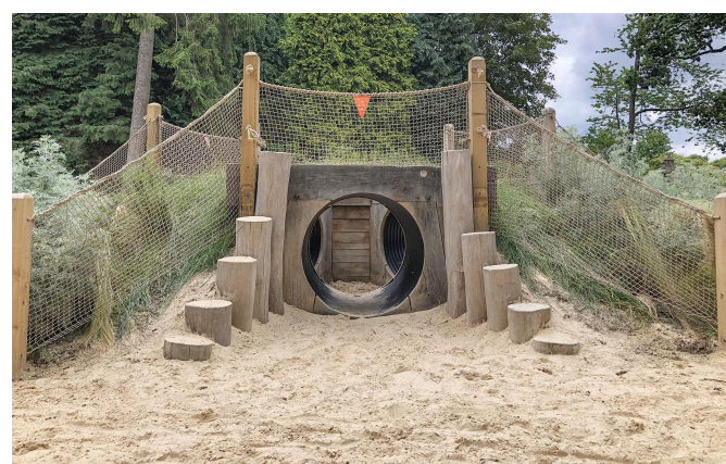
(C) Playground Tunnel
